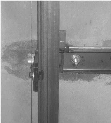
Leading rails installation on the rail fixing device
