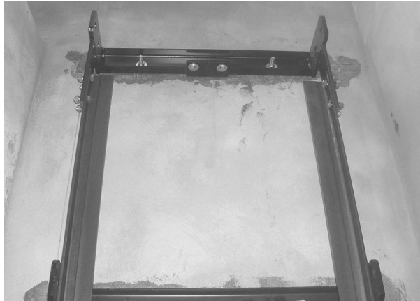
Leading rails installation on the rail fixing device
