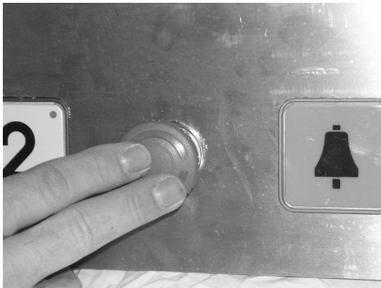
Emergency STOP button encroachment
