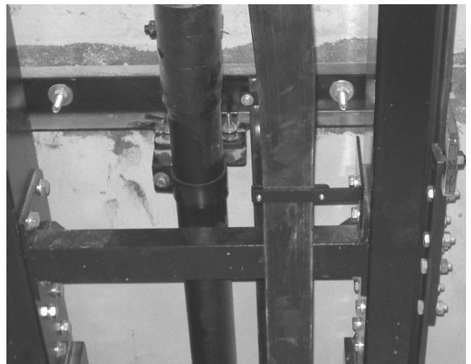
Ribbon cable fixing on the arcade
