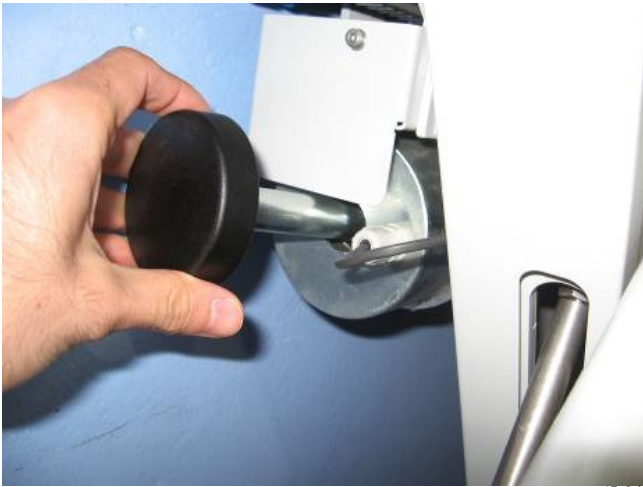
Handwheel insertion for manual handwinding of lift
